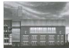
Trinity Middle School addition, Buttrick White & Burtis
